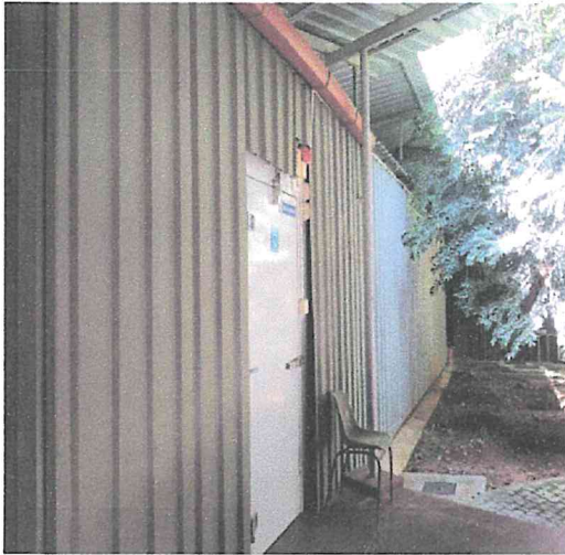
Cadaver storage facility
